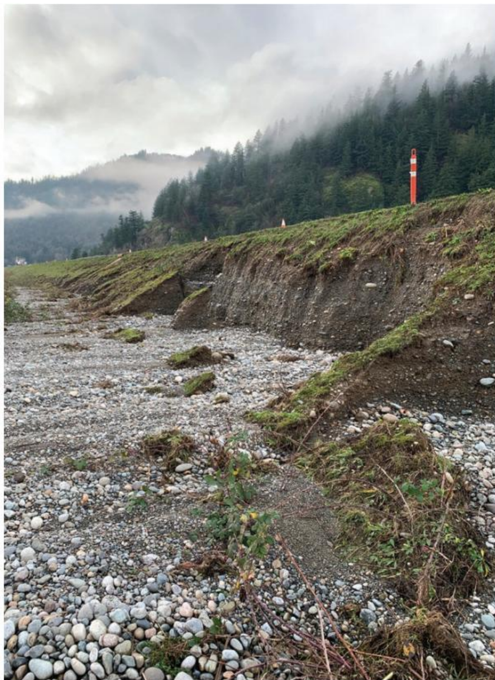
Figure 2. Erosion along the landside slope of the dike near the breach
