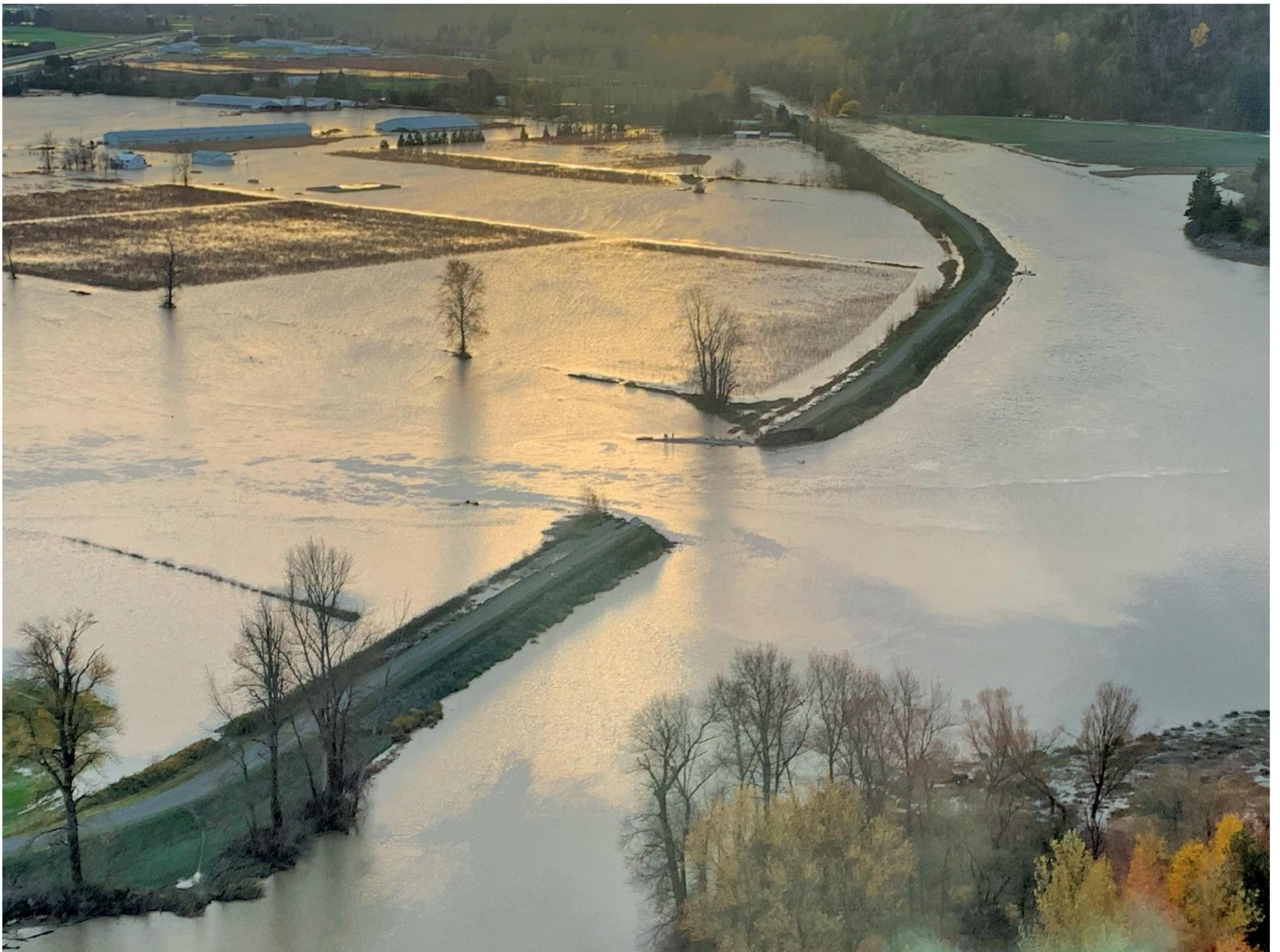
Figure 1. Sumas River Dike breach (water flow from right to left)
