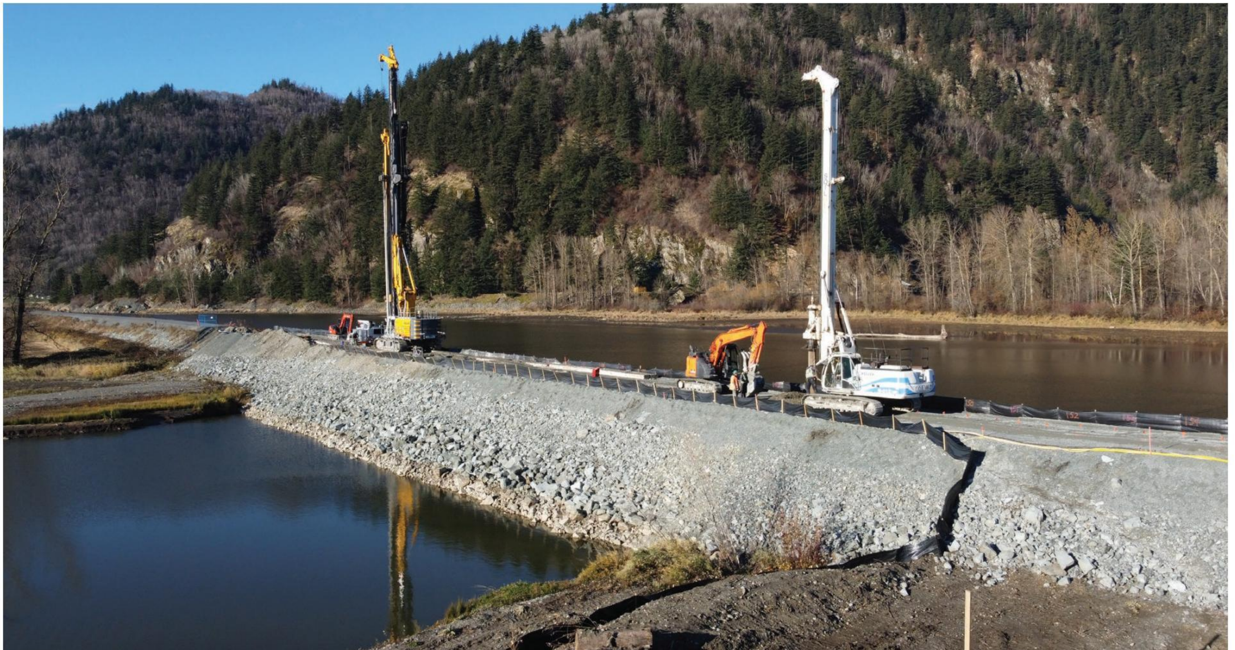
Figure 6. CSM rig and predrilling equipment on the dike breach closure
