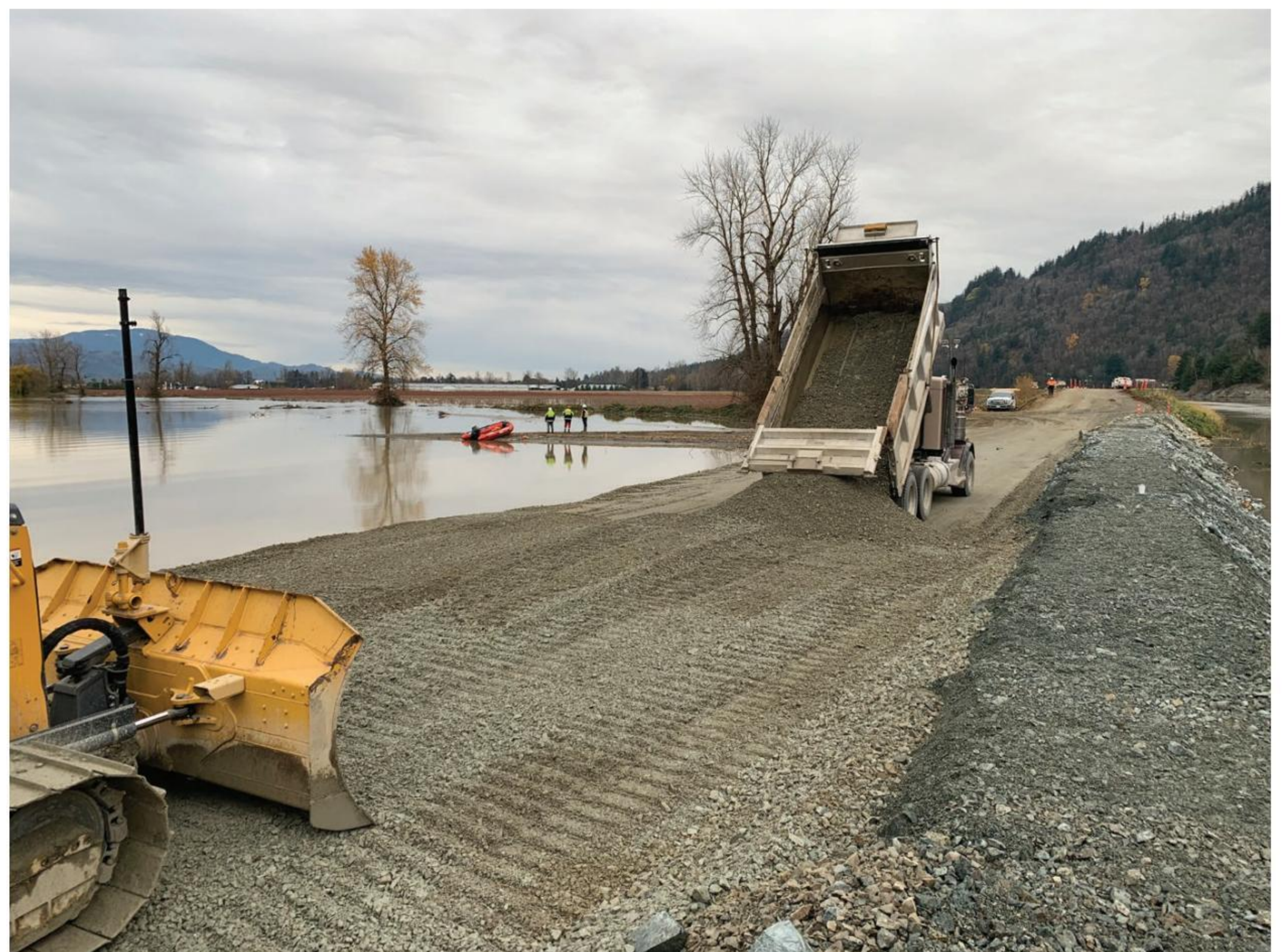
Figure 4. Constructing the central portion of the breach closure with finer crushed rock
