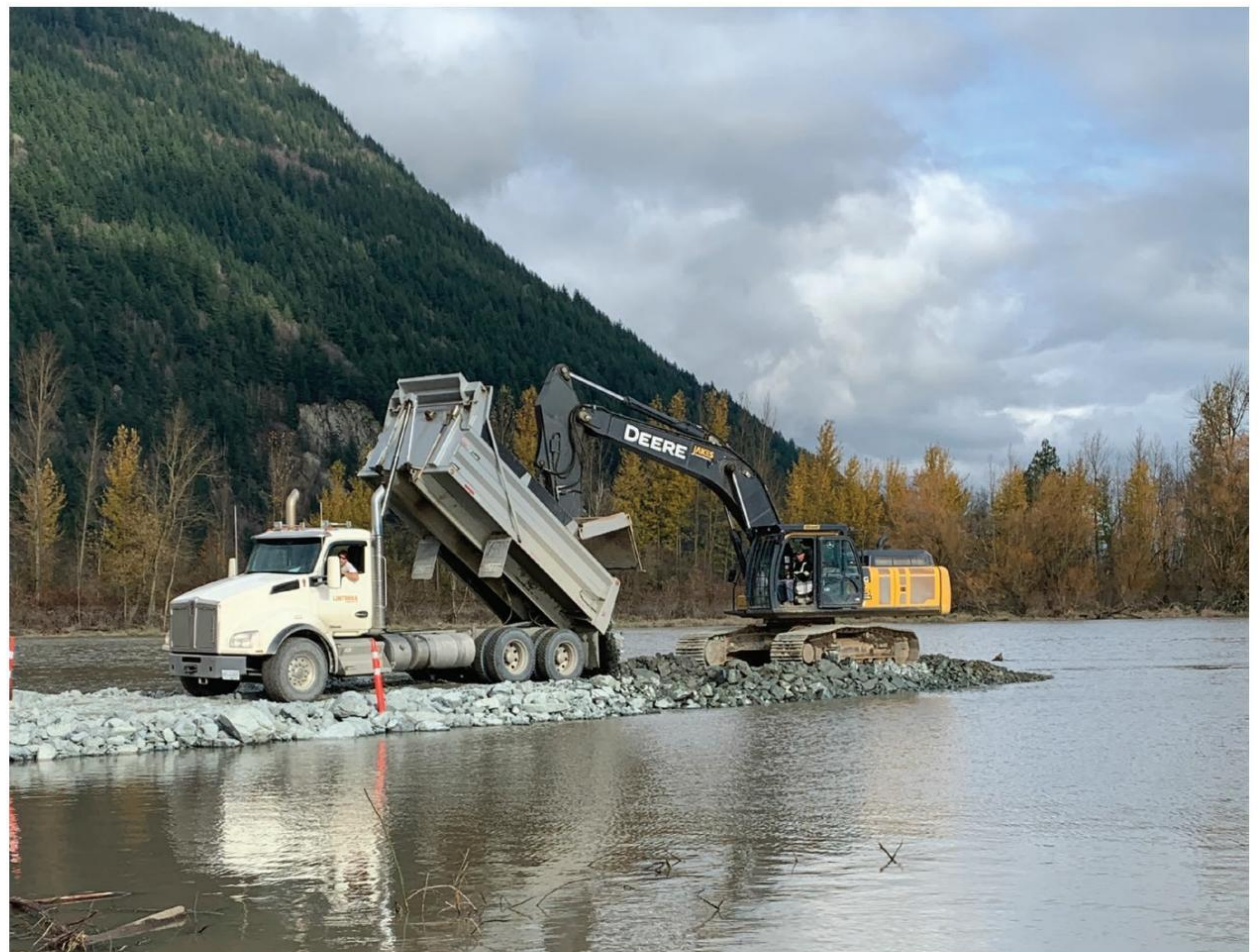
Figure 3. Initial emergency closure of the breach with coarser crushed rock
